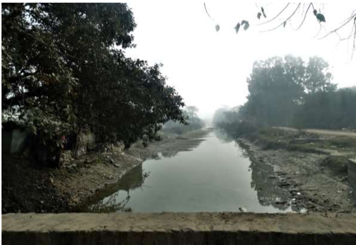
Image 32 : Upper Ganga Canal – Anupshahr Branch Near Unchagaon [Note the Siltation of the Canal]
